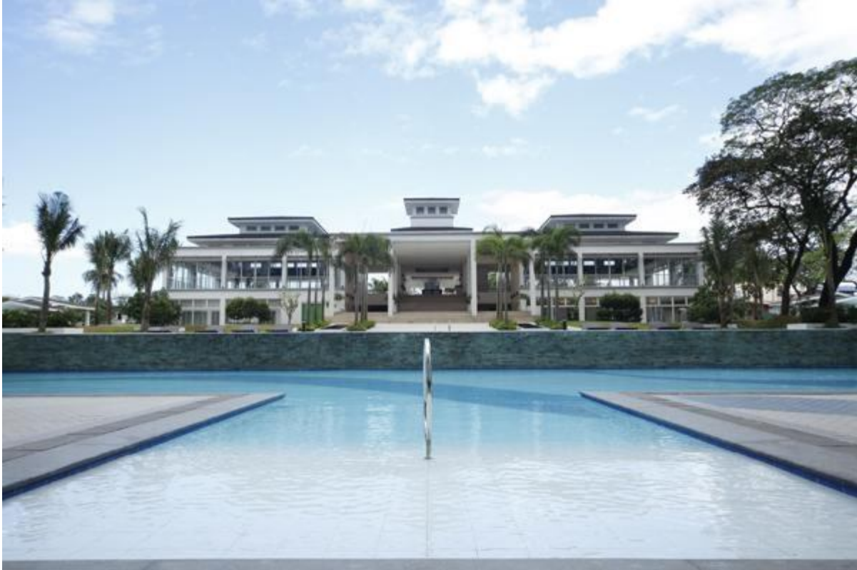
Grass Residences Clubhouse and Pool Area
